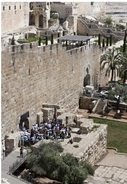
New gate drilled in the Old City southern wall
