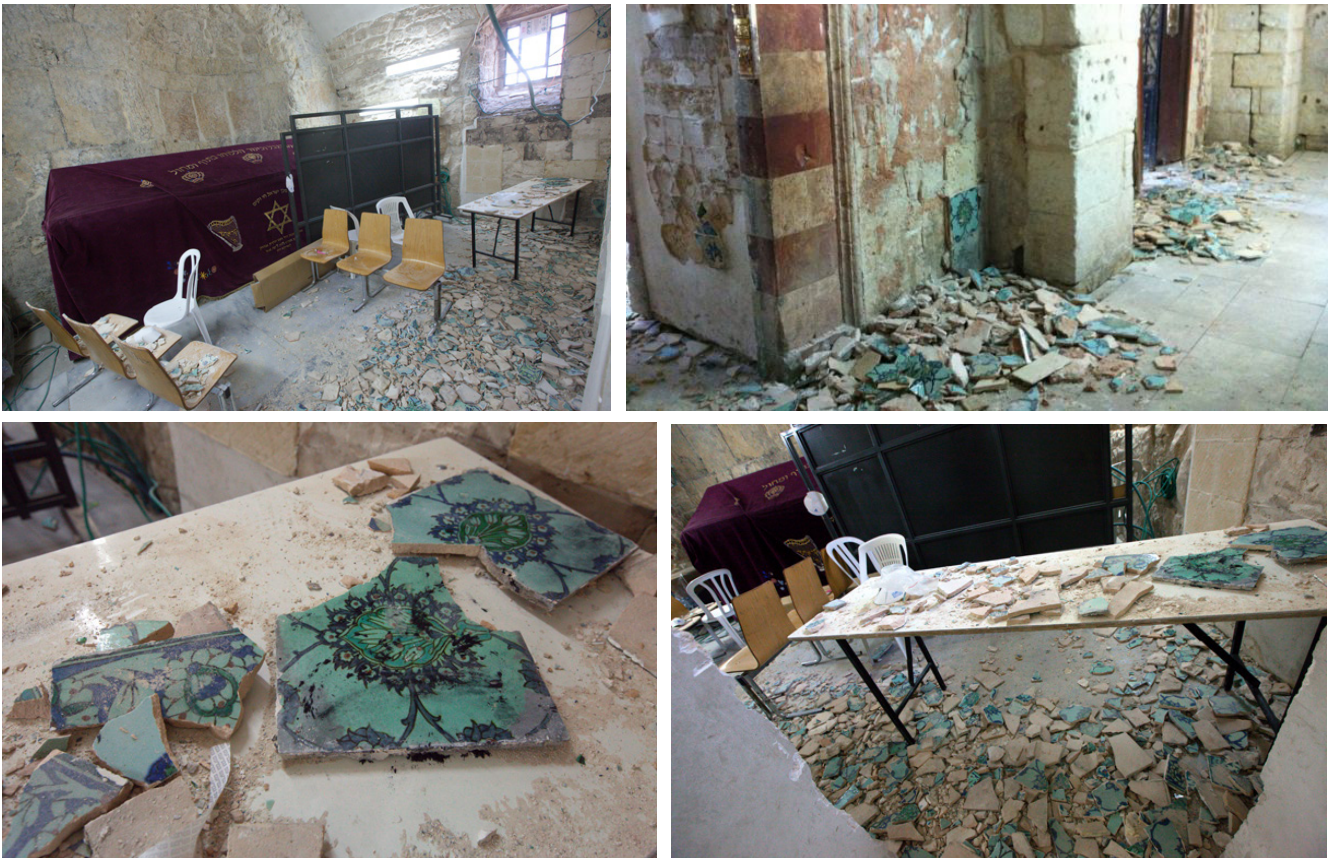
Documented damage at Nabi Dawoud Mosque.
